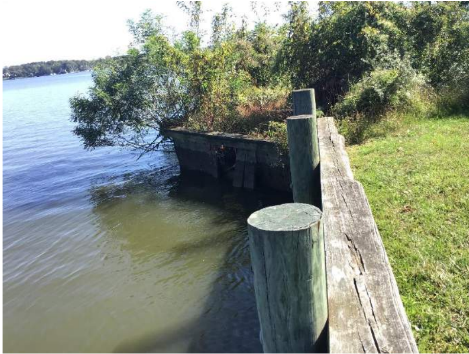
Photo 3: Failing bulkhead
