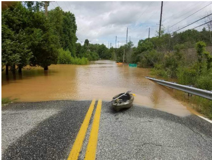
Figure 3: Photo of flooding from Peddlers Creek at Route 7 culvert
