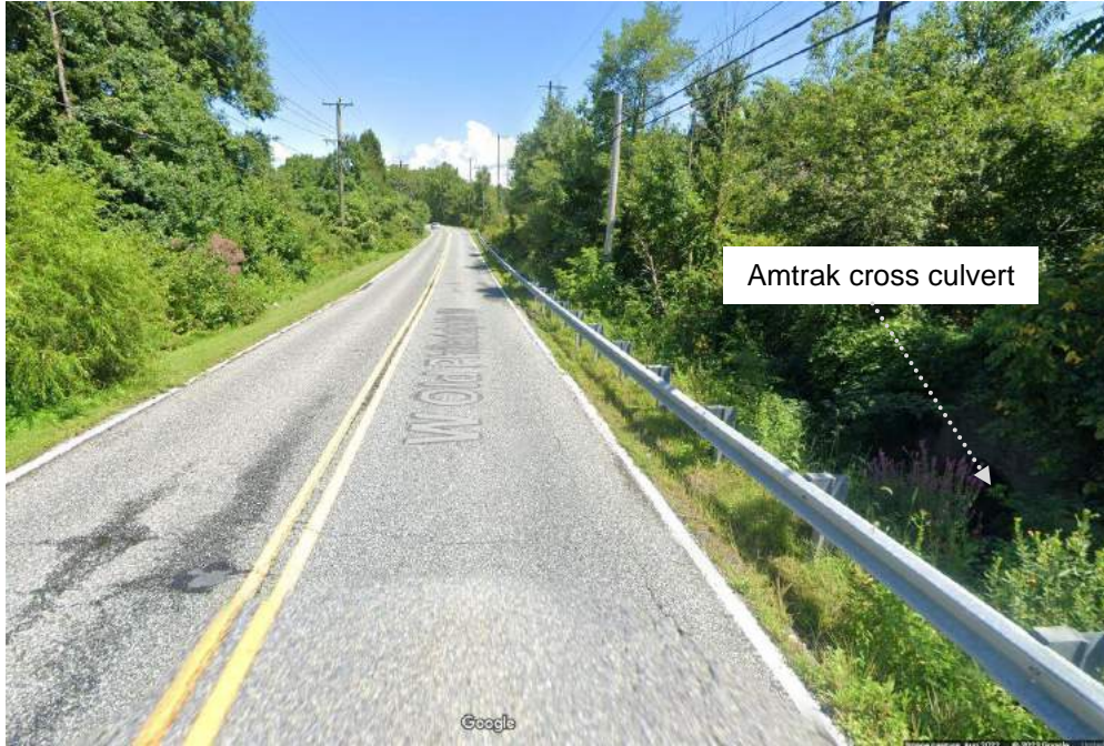
Photo 1: Peddlers Creek crossing at MD 7 and Amtrak cross culvert
