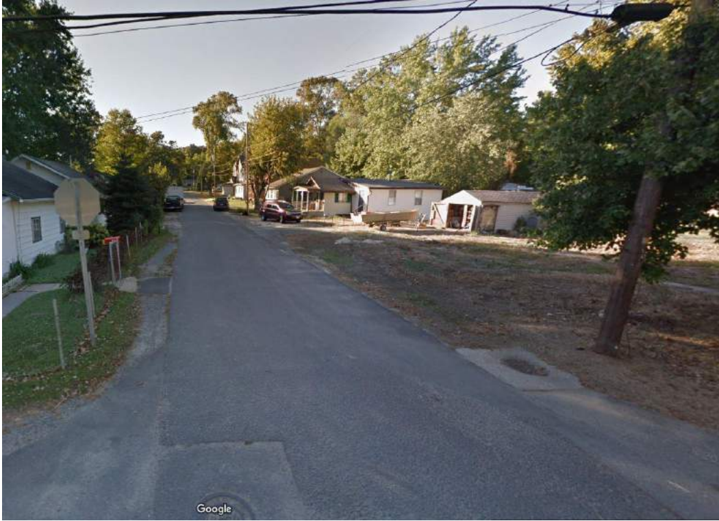
Photo 5: Chesapeake Road at Cecil Street intersection facing northwest towards Ogle Drive
