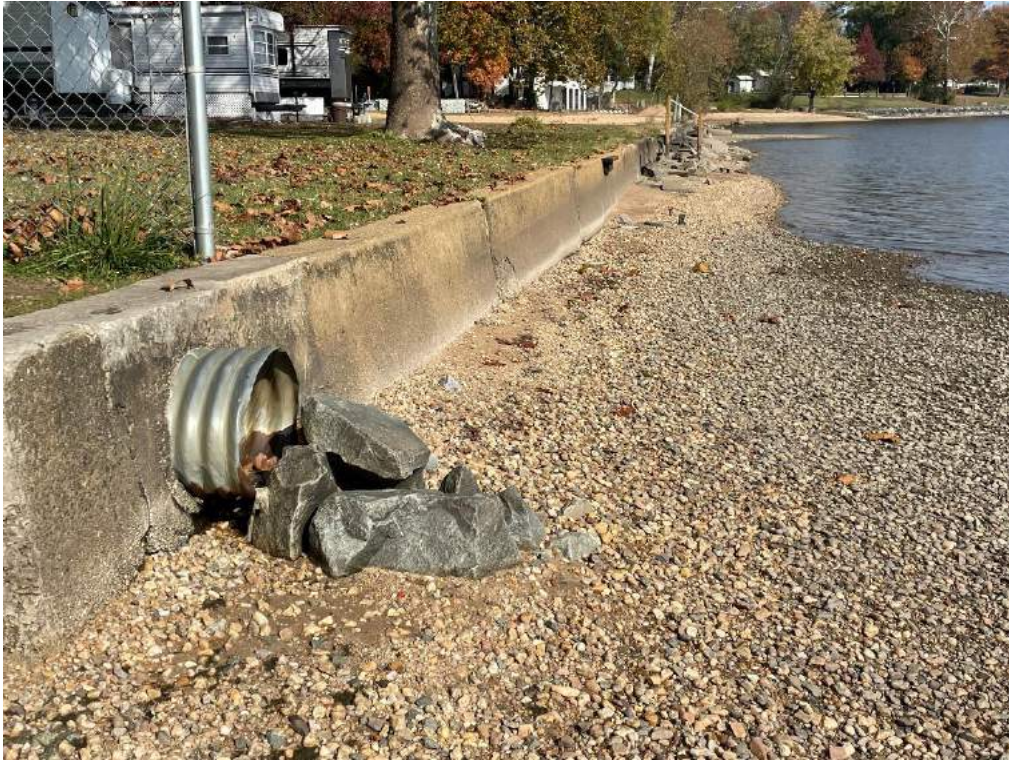
Photo 7: Outfall of Chesapeake Road storm drain system
