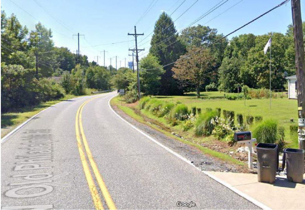
Photo 5: Roadside ditch which conveys runoff from MD 7 to Peddlers Creek
