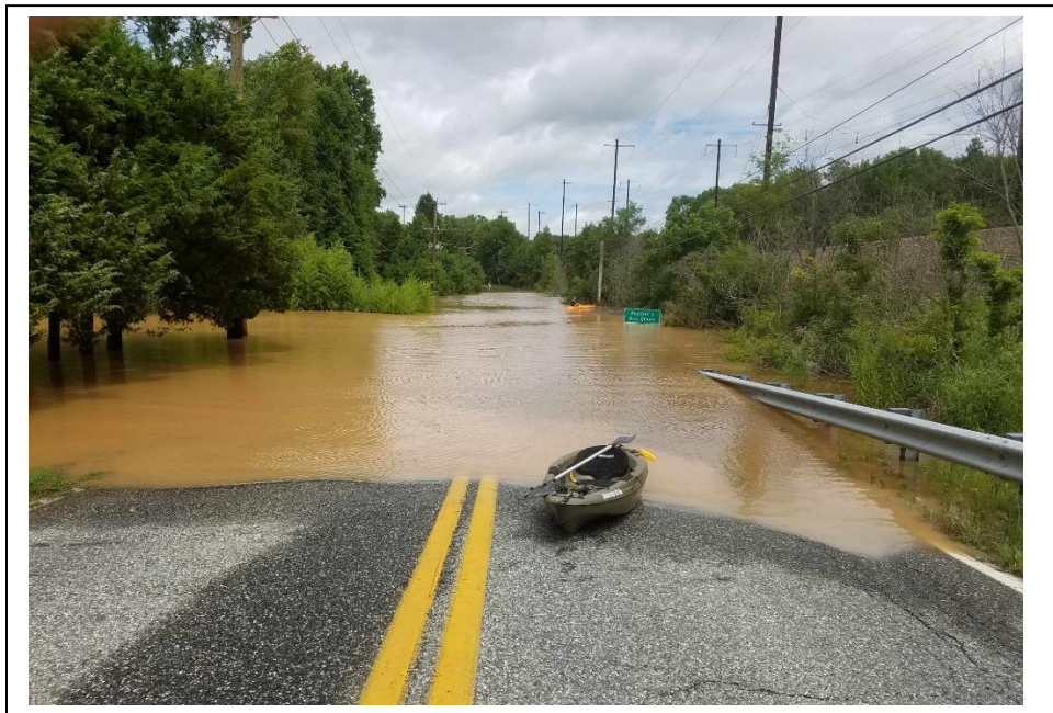
FIGURE 8: Photo of flooding from Peddlers Creek at Route 7 culvert
